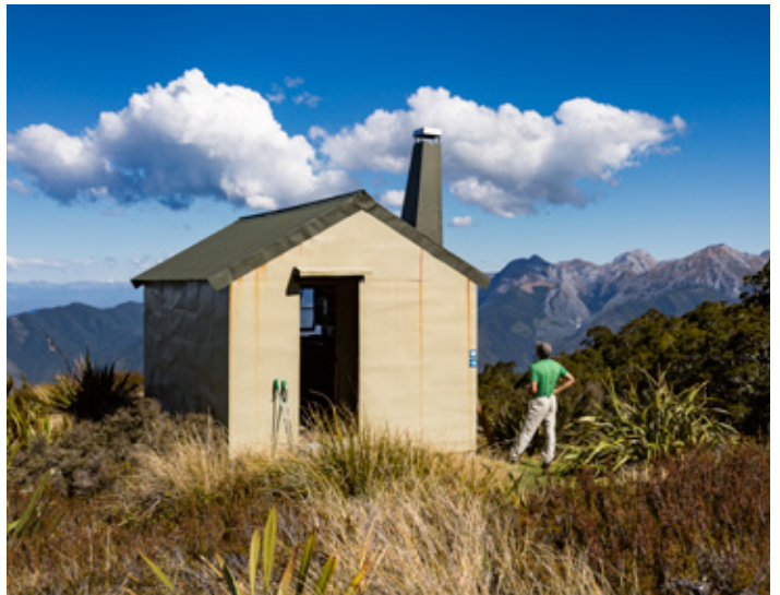
Silvano Lorandi sizes up the work needed on John Reid Hut
